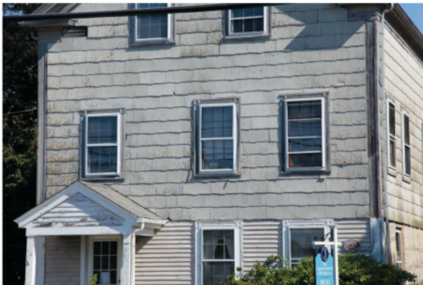
Figure 1. Before the renovation, the building was essentially sound, but the years had not been kind to it. Asbestos shingles covered the walls (left), and much of the trim had deteriorated beyond saving. As the exterior layers were peeled back, any of the original cypress trim that still had life was set aside to be reinstalled later (above).
